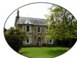
Victorian villa - 90 High Street
