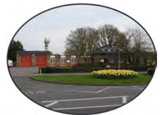
Fire Station on Ramsey Road
