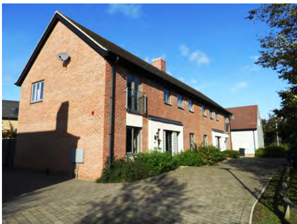
Lodge Drive exemplifies 21st century redevelopment of former industrial land within the centre of the village
