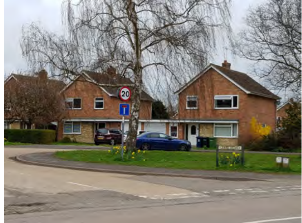
Two storey properties within Glebe Road with connecting flat roof garages and open space to the front where Glebe Road connects to Church Road.
