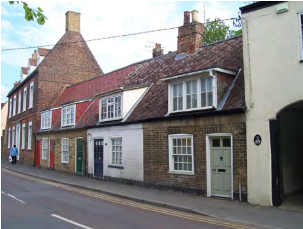
59-65 High Street demonstrating a continuous built form and variety of scale of development within the Historic Centre
