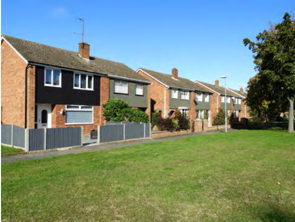
The semi-detached brick built houses with hanging tiles facing onto green open space in Booth Way typify 1960s homes growth in Little Paxton
