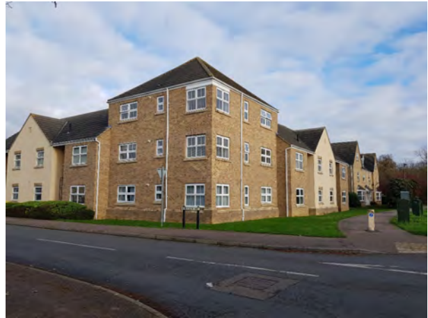
Flats on the corner between Robertson Way and Kings Ripton Road provide a distinctive landmark within this area and contrast between the mixed housing on Kings Ripton Road and the 21st century design within Robertson Way
