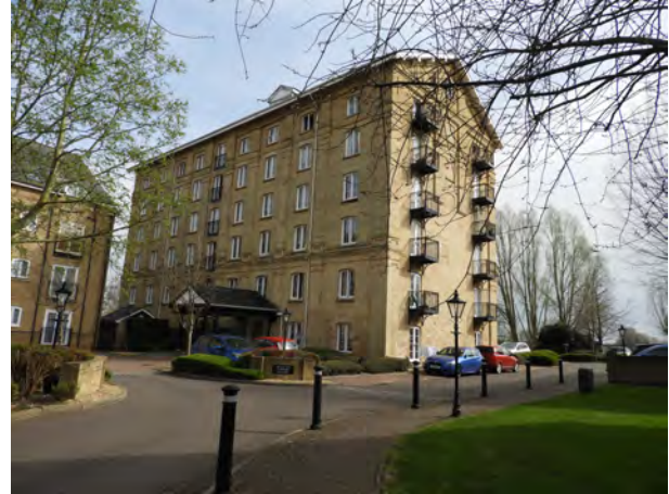
Riverside Mill has been converted into apartments
