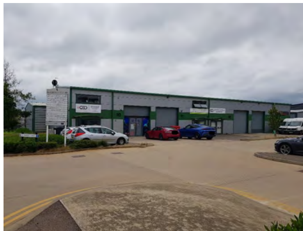
Enterprise Court within the Eagle Business Park
