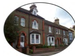
Hartford Road terrace
