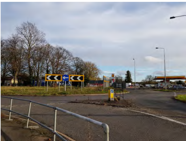
Buckden roundabout along the A1 forms a strong western edge to the village and separates Perry Road and Hardwick from the rest of the village with pedestrian access via two underpasses.
