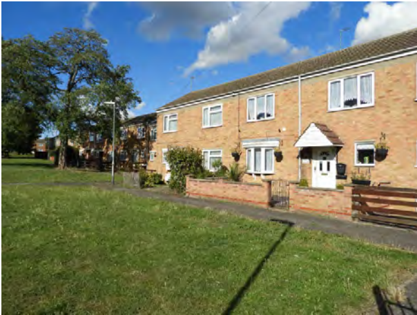
Kent Road shows the open space and pedestrian access to frontages common in the Radburn layout
