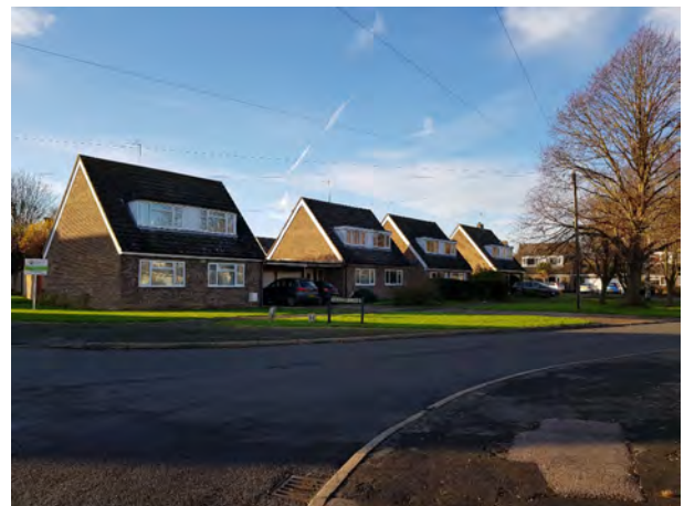
Aragon Close properties surrounding by open space and some tree planting. This is a common feature throughout the extensive residential aspects of the village although the design of houses vary
