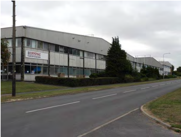
Large industrial units are set back behind grass verges containing mature trees
