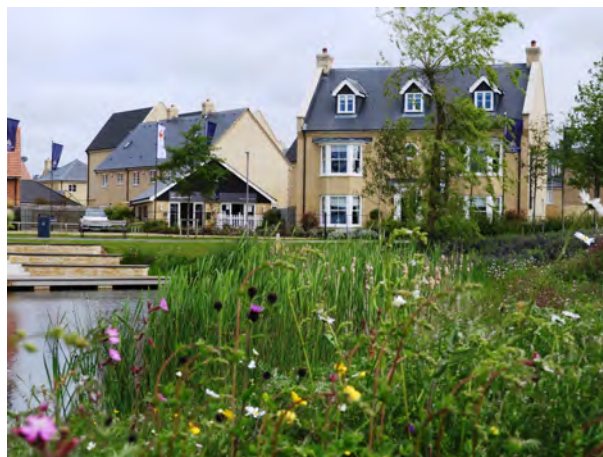
New homes, employment uses and community facilities are creating Alconbury Weald on the plateau formerly used for RAF Alconbury
