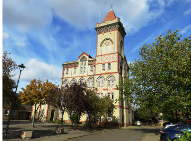
The elaborate brickwork and height of Paines Mill tower form a highly distinctive local landmark
