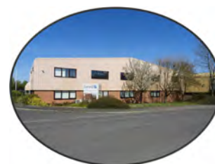
Landscape planting softens this industrial unit on Burrell Road
