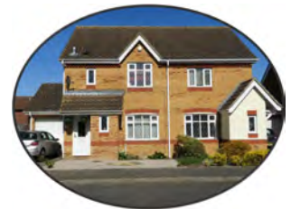
Different finishes help distinguish each house in the pair
