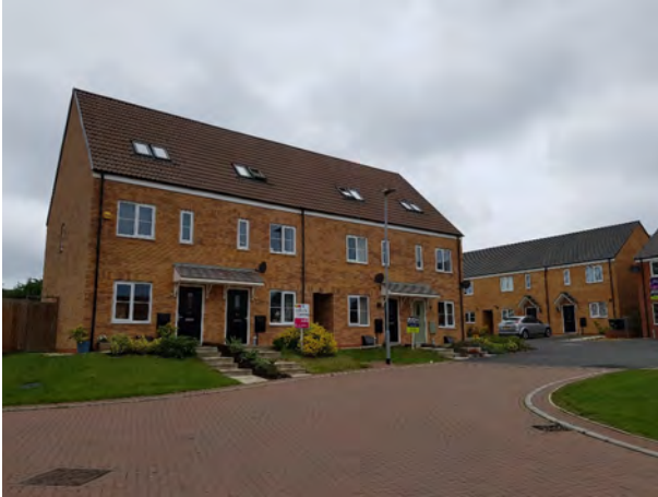
Terraces within Whitney Drive overlooking a central green space and areas of parking
