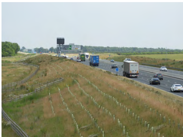
The A14 southern bypass cuts through the area adding extensive planting to soften the impact over time
