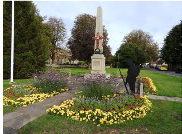
Eaton Socon war memorial is set in a substantial grassed area fronting Great North Road immediately south of St Mary's Church
