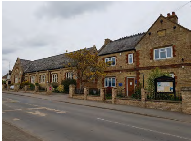
Old School Hall, Sawtry
