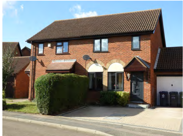
Further house type found and found across 'The Birds' estate in Sparrowhawk Way
