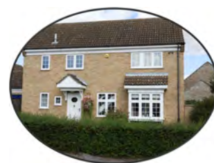
Buff brick house with box bay window and tiled porch features
