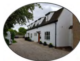
Modern infill on Church Lane
