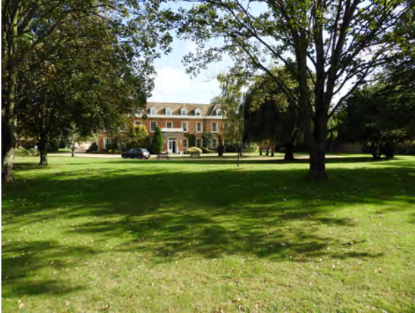
Paxton Hall originates from the mid 17th century with 19th century additions and built of red brick with limestone dressings. It is set in substantial landscaped gardens and is now used as a care home.
