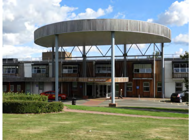
Hinchingsbrooke Hospital - civic buildings set in open landscaping
