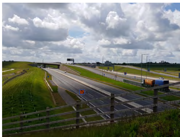
View of the A1 and A14 from overpass looking southwards
