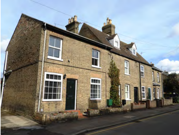
The mixed heights of properties along East Street add variety to its character
