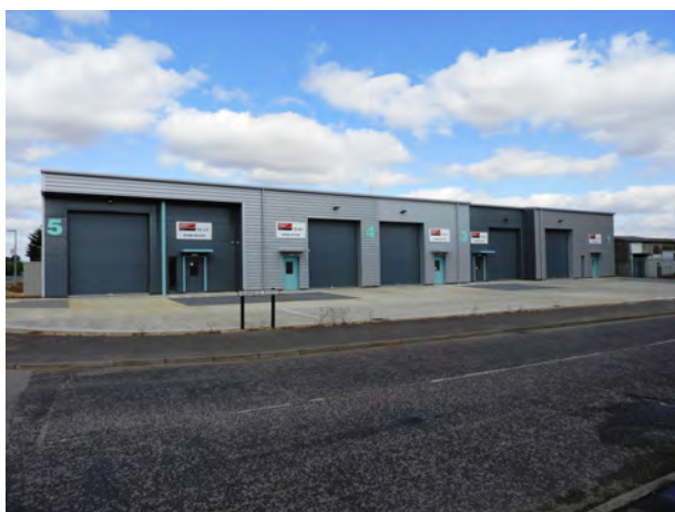
Simple structures in soft grey and neutral shades typify more recent industrial buildings
