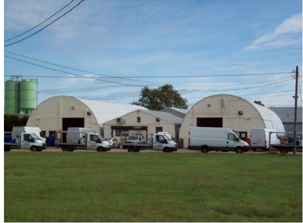
Some original military buildings remain at Little Staughton Airfield but most is now used as a solar farm
