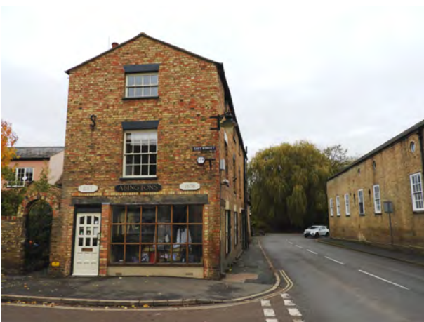
Sharp bends affects the eastern approach into the historic centre
