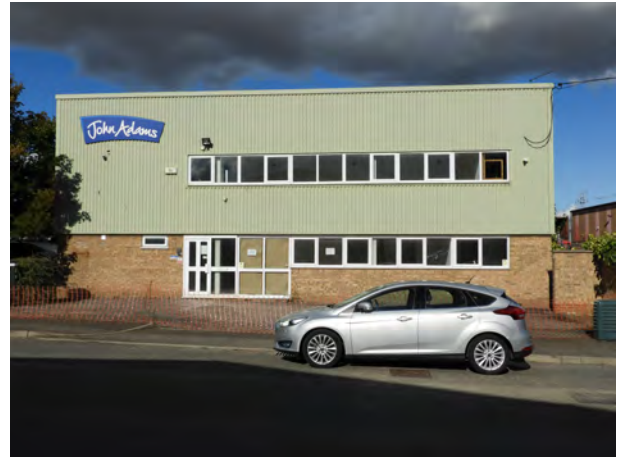
Alms Close - typical blending of brickwork and steel cladding
