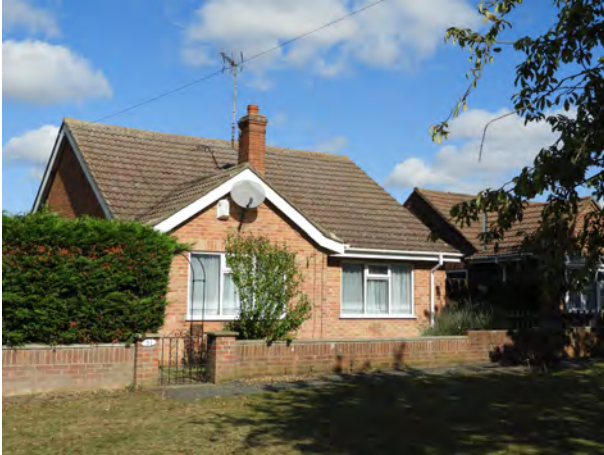
This bungalow on Arundel Road is typical of many in the immediate locality forming an area of relatively low density housing
