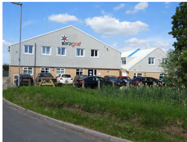
Unit within the West Newlands Industrial Estate constructed from a mixture of buff brick and cladding
