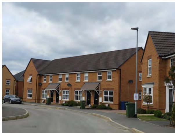
Example of terraced development along Saxon Close within phase 2 of development
