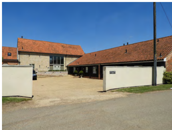
Manor Farm Court , Great Haddon is an example of successful barn conversions
