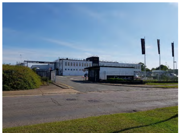
Hotel Chocolat located within the St Peter's Industrial Area it is one example of industrial units within Huntingdon. Huntingdon has several industrial areas located on the edge of the town and are key sources of local employment.
