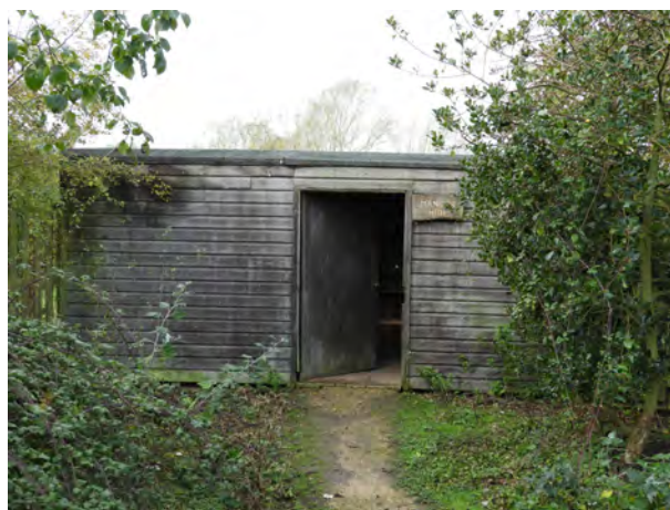
Mander Park bird watching hide provides an opportunity for people to interact with nature without causing disturbance; the wooden building blends well into the surrounding trees and shrubs minimising its impact on wider views
