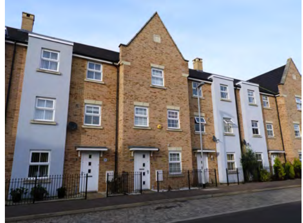
Three storey townhouses in Buttercup Avenue are designed to make efficient use of land
