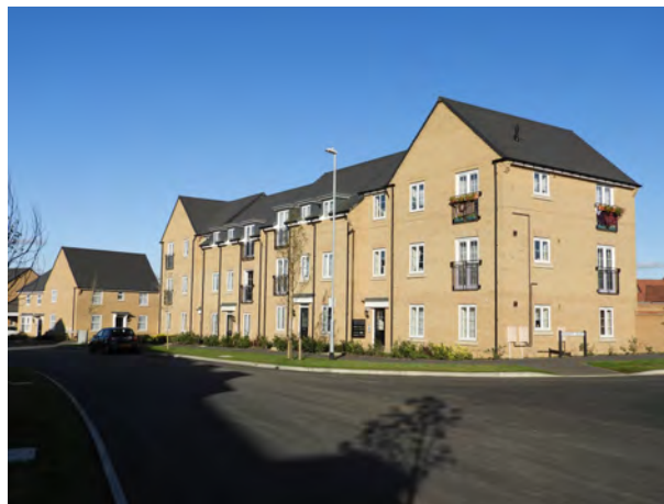
Three storey properties give variety and definition along one of the main roads within Romans' Edge and help to enclose the streetscene
