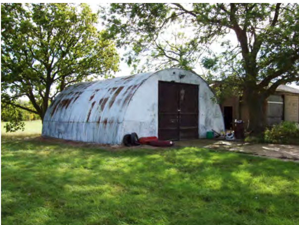
Little Staughton airfield nissan hut
