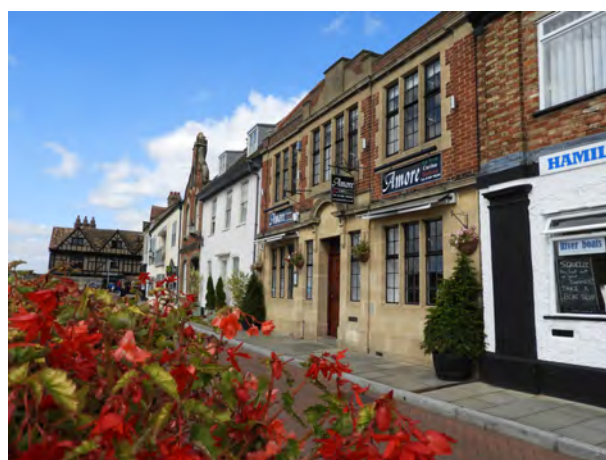
Quayside buildings reflect St Ives' important river trading history
