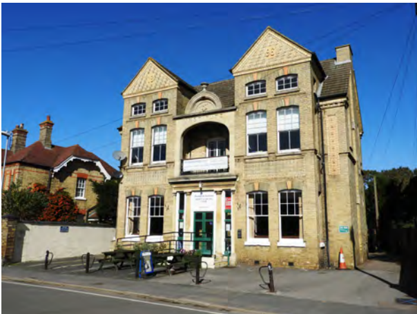
Brampton Institute, Brampton
